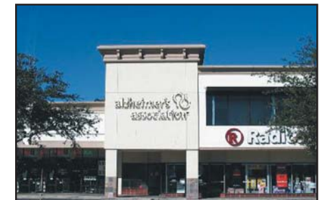
The new home of the Houston and Southeast Texas Chapter of the Alzheimer's Association.
